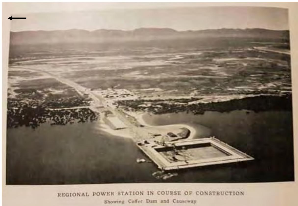
Figure 5.1: Playford A Station foundation construction, circa 1950's (FPP)
